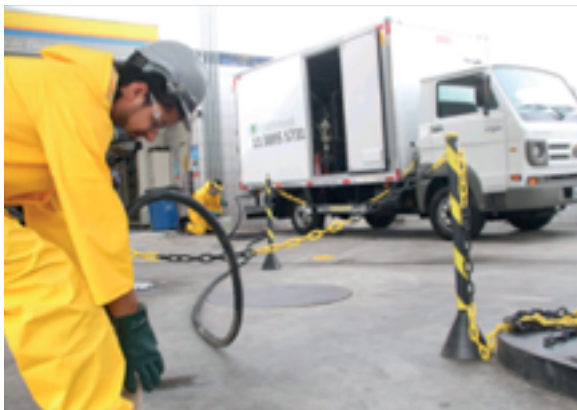
Injection - System Redentis / Fentox in Operation
